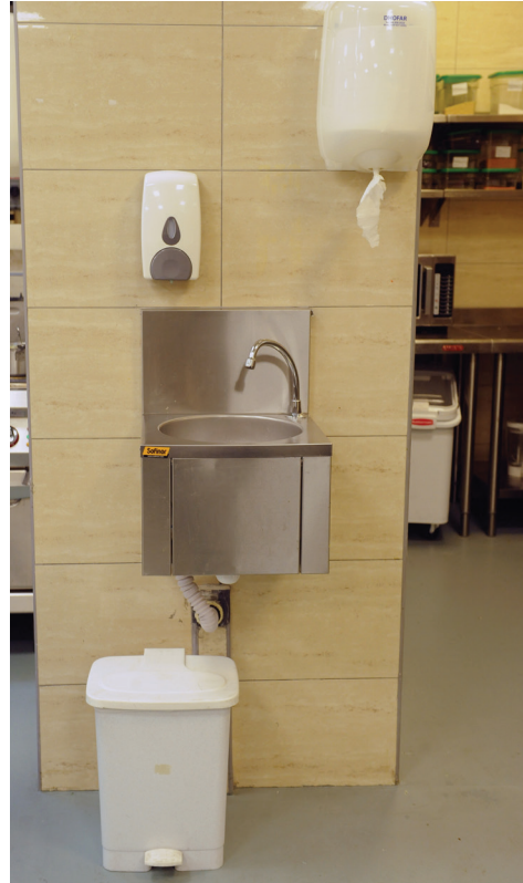
figure 5:well maintained walls
